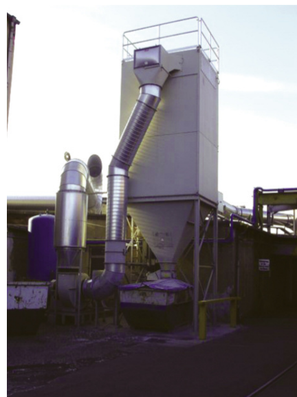
Centralized filter with constructive explosion protection
