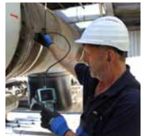
Getting an insight into the interior of the ductwork by endoscopes
