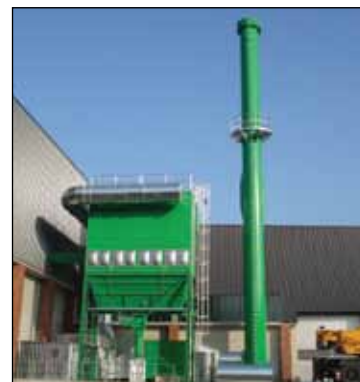
Filter unit with burst disks
